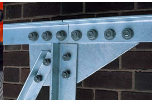
Sherardized fasteners in building steel work construction. 4.6, 8.8 and 10.9 grades of fasteners can be treated without affecting their properties.
